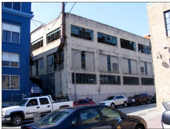
Warehouse space slated for demolition. Image Source: Brent Beane on behalf of ULI Washington.
