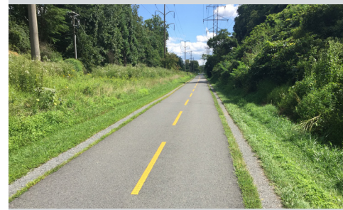
Bluestone areas along the edge of the trail should be maintained and expanded to allow joggers to use these areas. Source: Schwanke.
