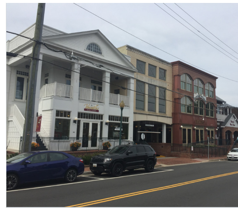
Improved connections between the Town and the trail will boost economic and pedestrian activity in the center of town, enriching the heart of the community. Source: Schwanke.
