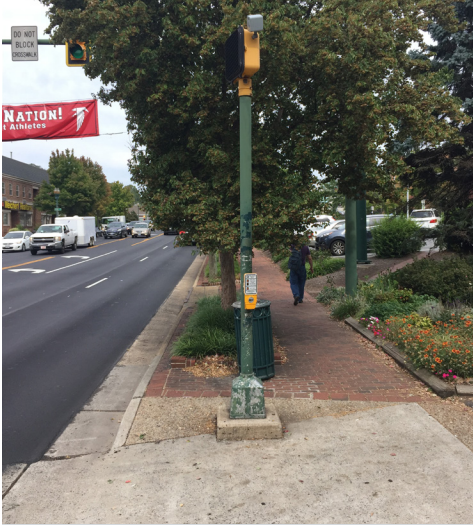
The signal button the east side of Maple should be moved back from the street to increase pedestrian safety. Source: Schwanke.
